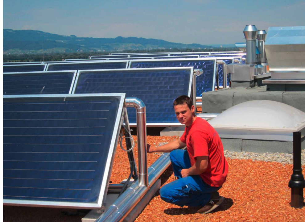
A photovoltaic roof application by the village plumbers
